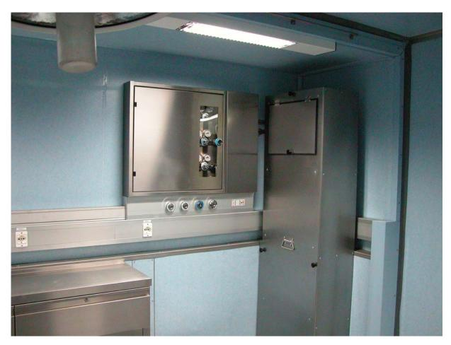
The system is composed by a general gas plan with pressure reductions and gas alarm complied with the medical regulations.
